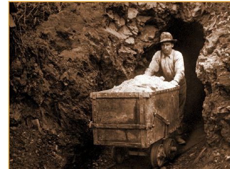
Mount Sicker's Lenora Mine - tunnel #1
