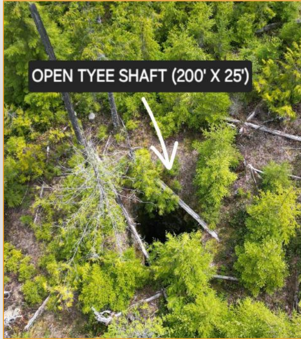
Open shaft hidden by trees, 25ft across and over 200 ft deep
