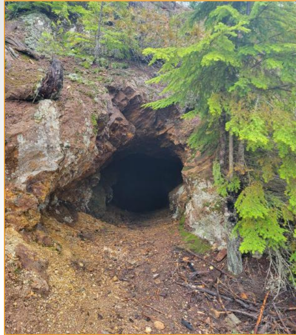
Open adits all over the area - to be sealed with special screens*
